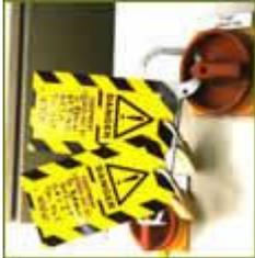
If the electrical power has been turned off to allow you to do work safely, it is essential that the power stays off until you have finished work. Make sure YOU are in control and STAY in control. A good way is to have the only key to the switch or a locked room or cabinet containing the switch. Remember, if you remove a fuse, another one could be inserted in its place, and people ignore notices. If you have any doubts that the electricity may be turned on again without you agreeing, STOP WORK.
