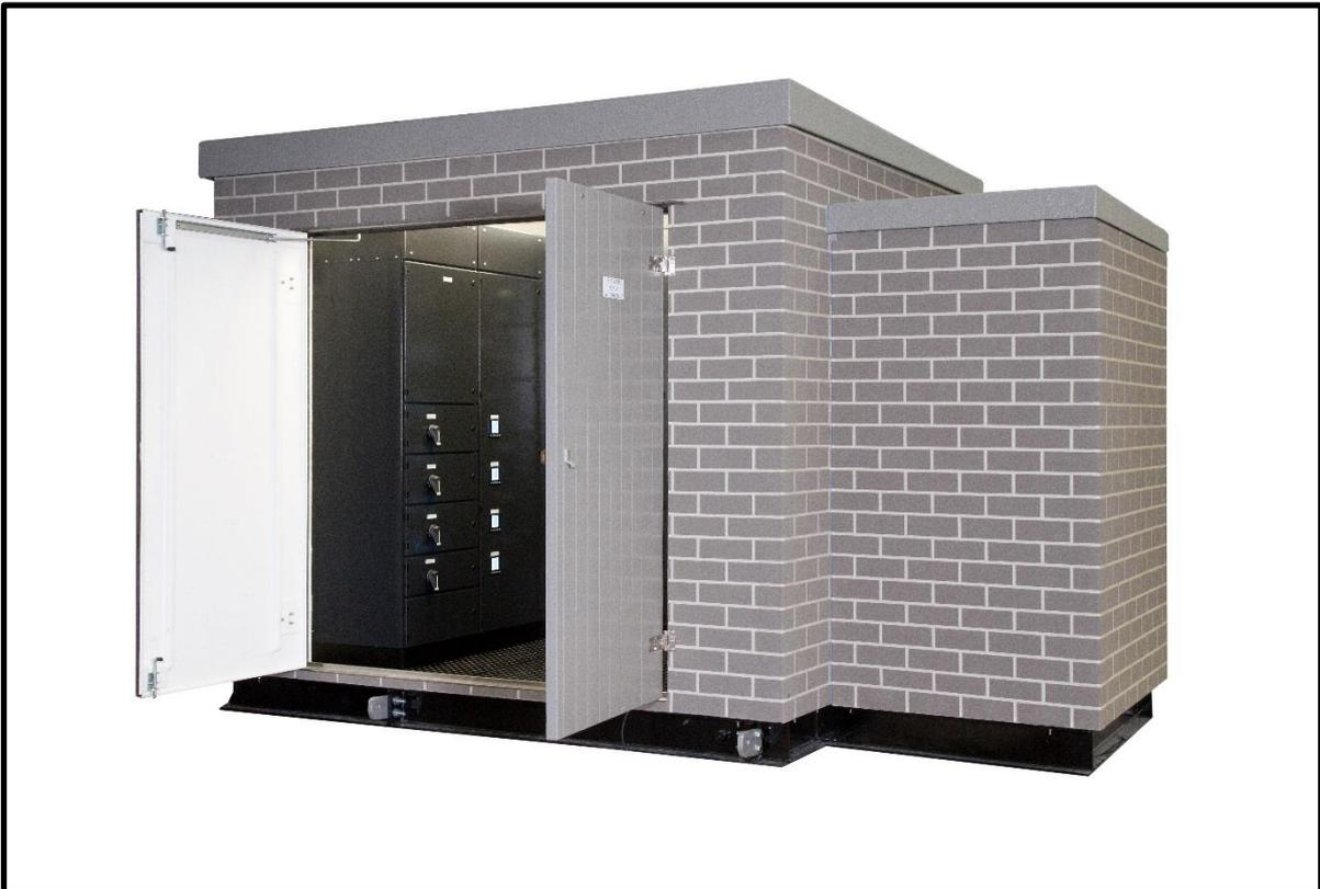
The low voltage switchboard housed in a GRP enclosure – pre dispatch.
